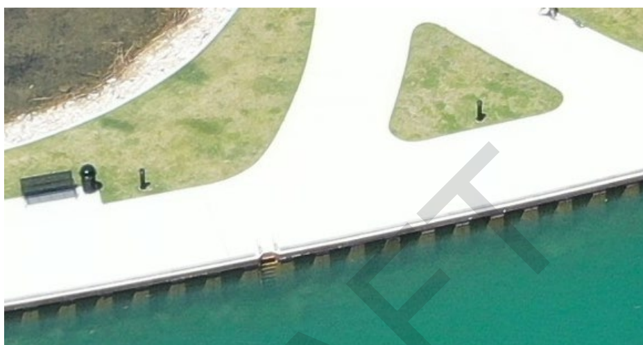
Figure 6. Sheetpile face with concrete decking.
