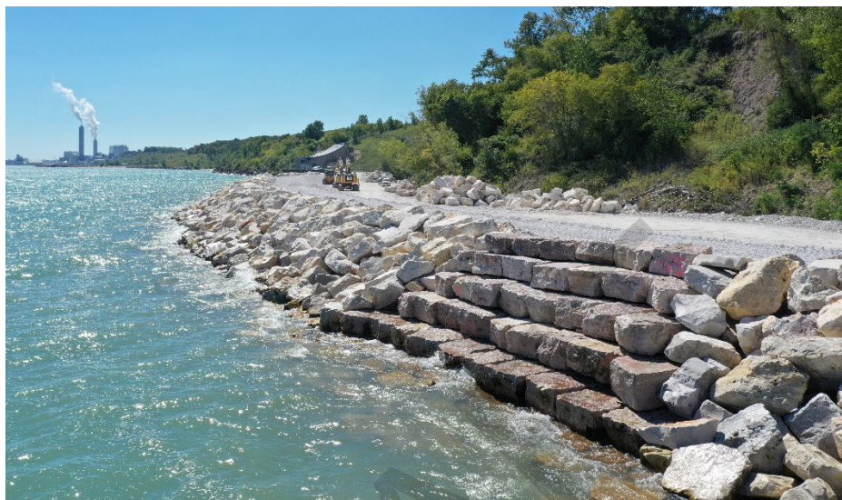
Figure 7. Terrace stone water touch point included along a revetment.
