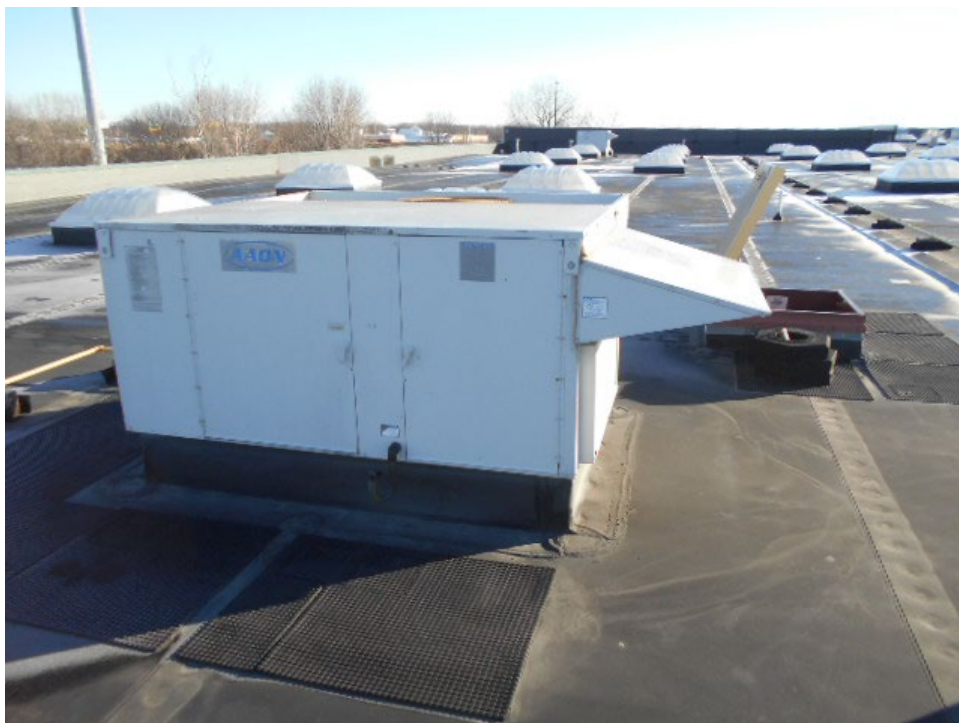
Subject Roof HVAC
