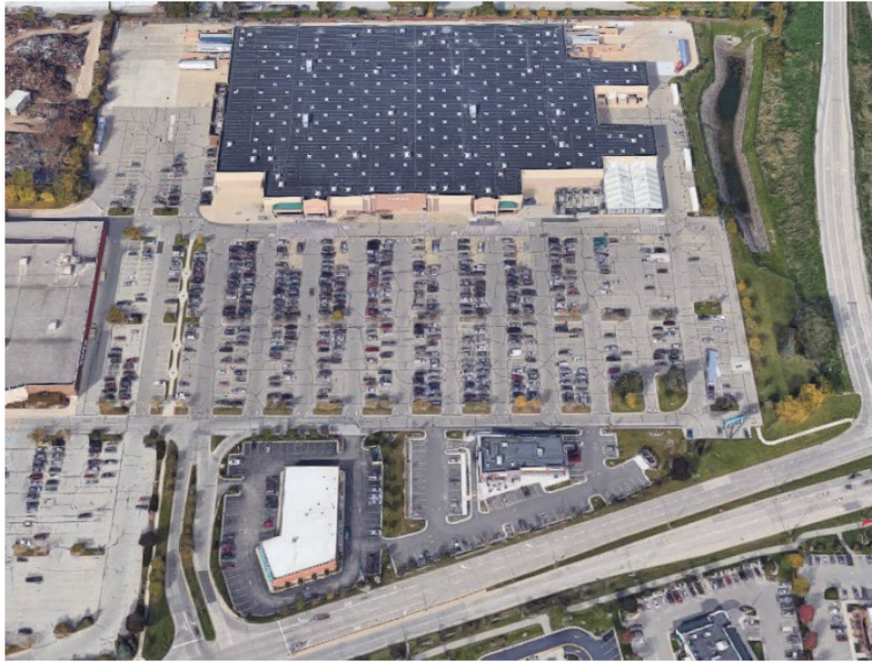
Bird's Eye View Facing West
