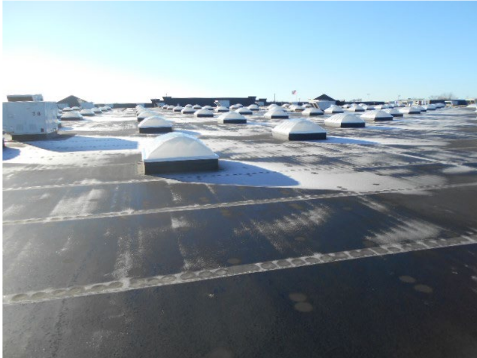
Subject Roof Cover and Skylights
