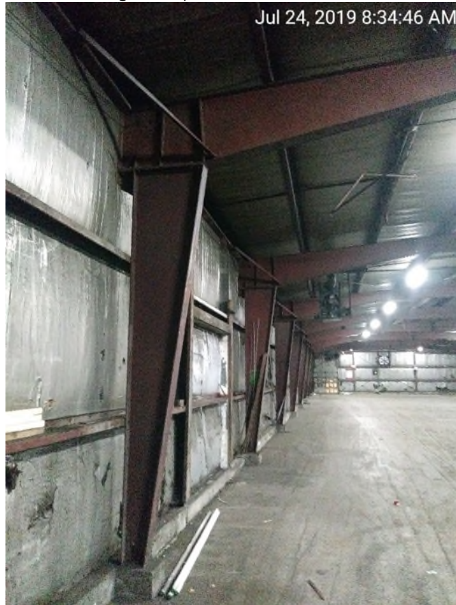
Warehouse – Interior (East wall looking south)
