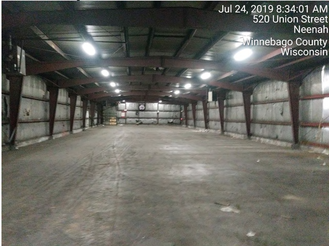
Warehouse – Interior looking south
