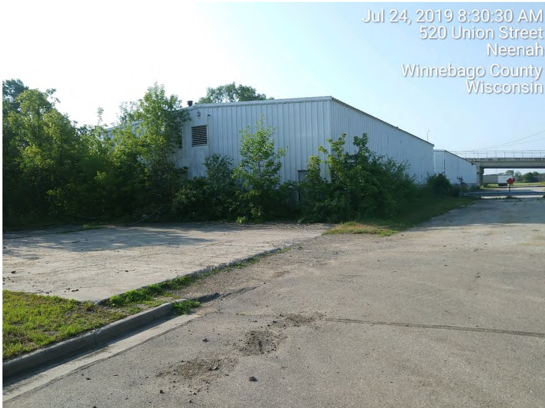
Warehouse – North face
