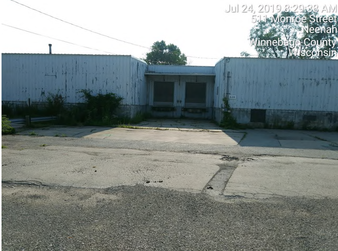
Warehouse – Loading dock area
